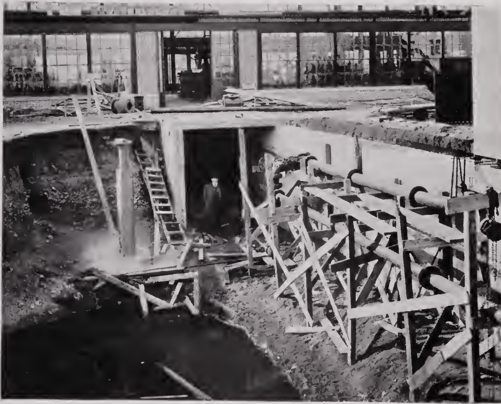
WHERE WATER SUPPLY IS LOCATED Forge Steam Plant to be Fed From Underground Tank
